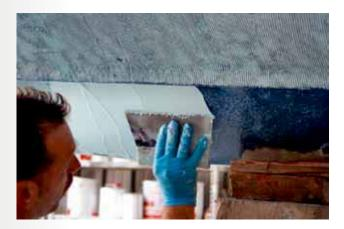
8 Sanding of the whole hull with 60 grade abrasive paper.
