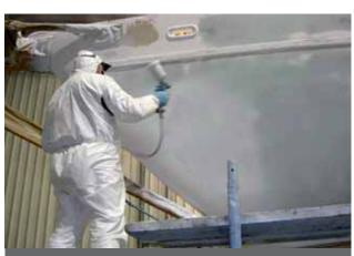
Areas not to be painted and those requiring a different paint system shall be masked. Spraying is a very effective application procedure but requires a professional operator.
